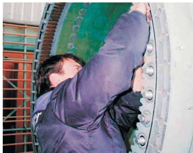
Figure 2. The bolting on a rotor blade bearing of a modern wind turbine. Picture: August Friedberg GmbH
